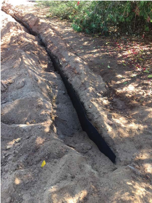
Root Deterrent installation at Sandalwood Arts
