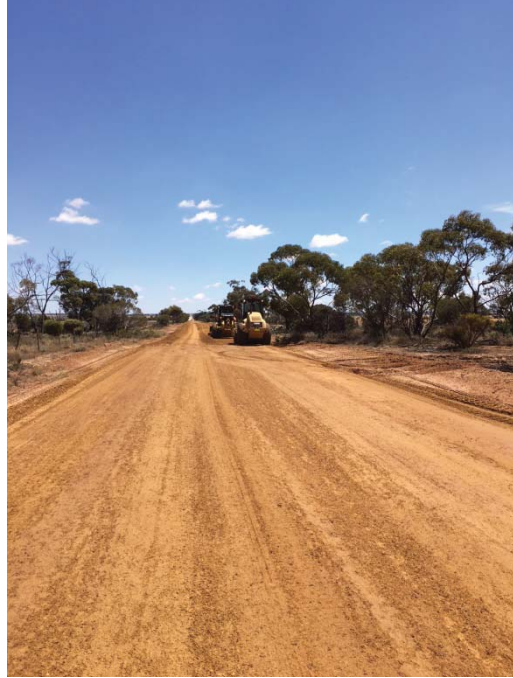
Barbalin North Road Construction
